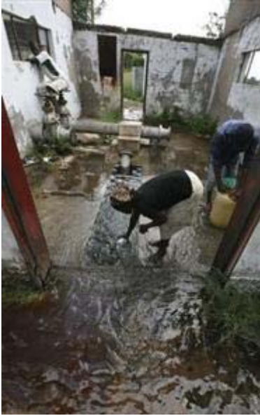
Residents fetching water from burst pipes
